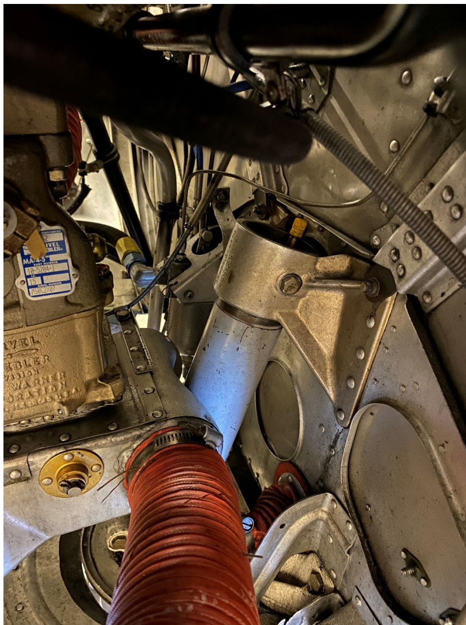
Photo 3 – View of the firewall on accident airplane at the Elmendorf Aero Club’s hangar. Photo provided by the FAA.
