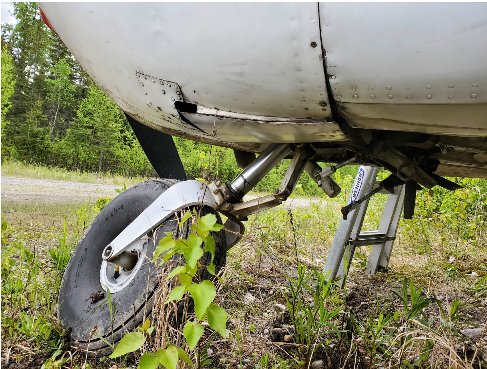
Photo 2 - Damage to firewall. (Photograph courtesy of the airplane owner.)
