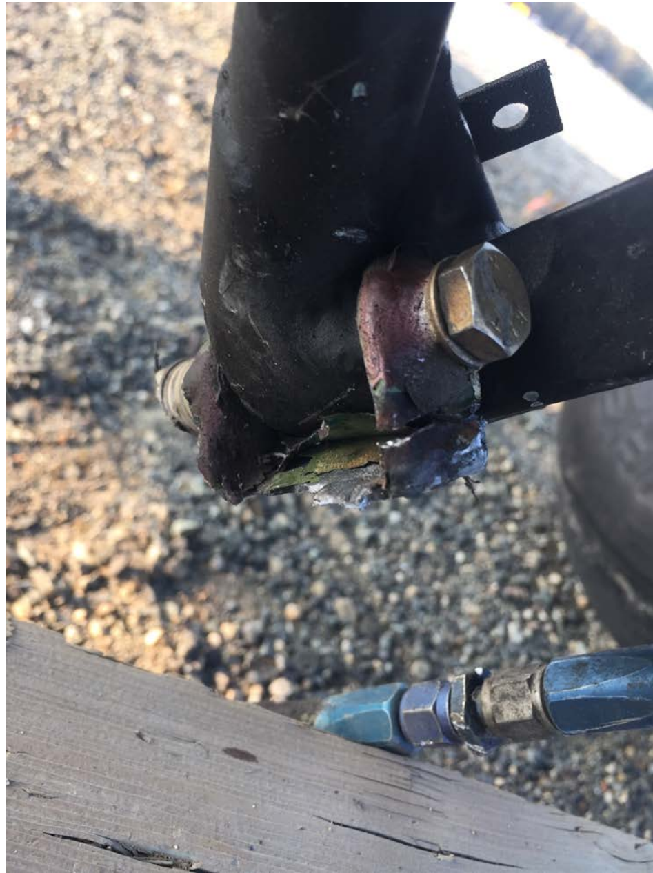
Photo 2 – Landing gear with separated landing gear fitting attached.
